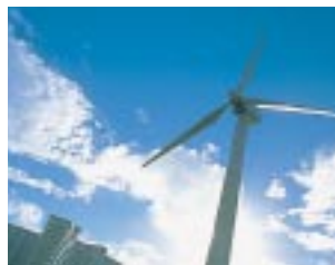
Okinawa Zanpamisaki Royal Hotel has cut its electricity bills by around 15% through the use of in-house wind-powered generation facilities.
