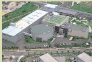
Daiwa House Industry's Central Research Laboratory consists of the Main Building, the Techno Laboratory and the Experimental House.
