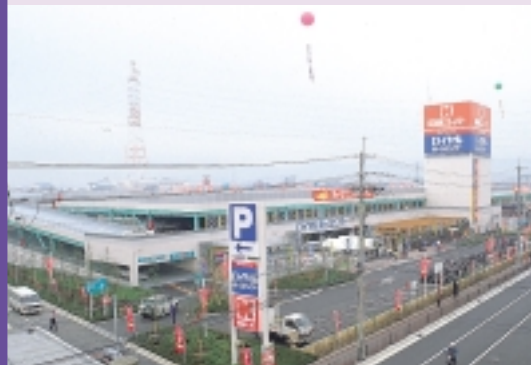
◆Royal Home Center Nishikanmuri in Osaka Prefecture.
