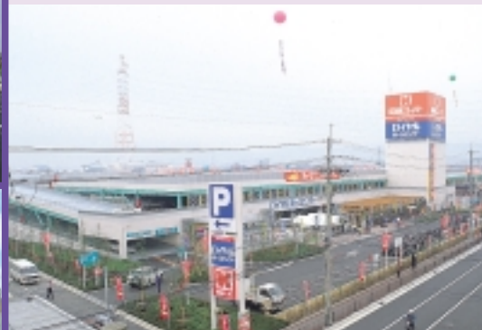
◆Royal Home Center Nishikanmuri in Osaka Prefecture.
