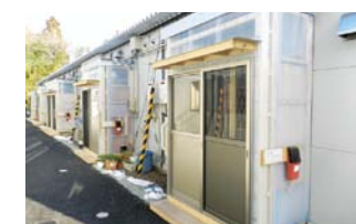
Windbreak porches installed in front of the entrances
