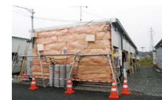
Double-layering of end-walls and double-glazing work
