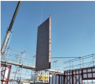
Exterior drywall panel (Installation)
