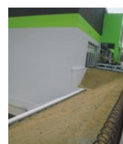
Part of the building submerged under the ground to improve heat insulation
