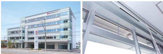
Daiwa House Fukushima Building, which adopted a passive air flow window
