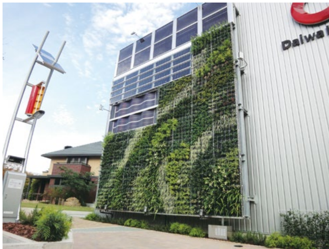
A building installed with the air-purifying wall greening system (D-room Plaza Hall of our company)
