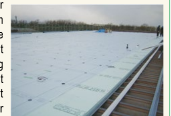
Renovation for heat insulation of the roof
