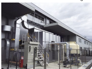
Combustion exhaust gas treatment device with thermal storage
