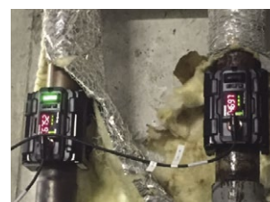
Measurement using flow sensors
