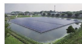
Floating solar power plant on reservoir (Daiwa Lease)
