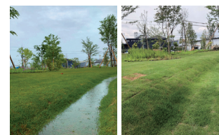
Rain garden (Left) During rain (Right) Rain water infiltration after rainfall
