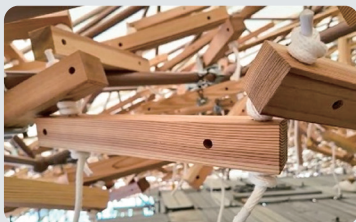
Wooden inside-roof members rope-secured to facilitate reuse
