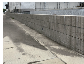
Flood countermeasures: Raising waterway boundaries
