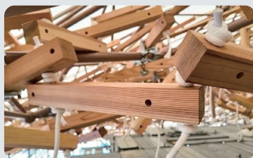
Wooden inside-roof members rope-secured to facilitate reuse
