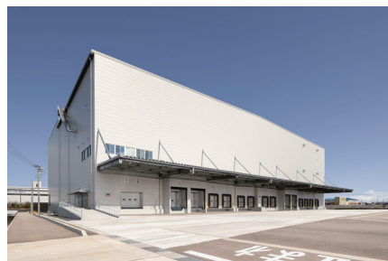
Wakamatsu Konpou Unyu Soko's Head Office No. 2 Joint Distribution Center (Ishikawa Prefecture)
