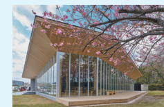
Dining hall in Kawamura Electric Inc.'s Tsukuba Plant (Ibaraki Prefecture)
