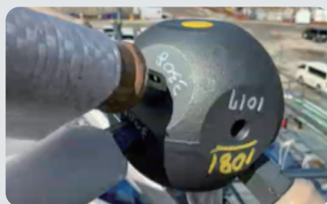
Components part and assembly-sequence numbered with indelible paint to enable easy reassembly
