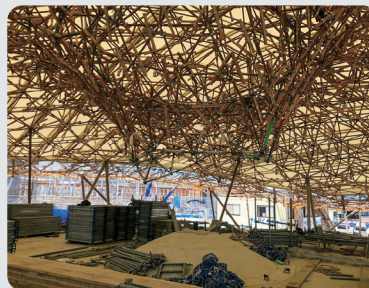
Assembly done while referencing over 1,000 drawings to allow for gravitational forces not in the drawings
