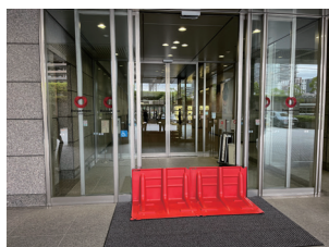
Water barrier at the Osaka Head Office
