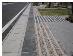
Adopting green infrastructure principles: Gravel laid within green blocks
