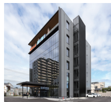
The SHOWA CONSTRUCTION Co., Ltd. head office building (Fukuoka Prefecture), an office that achieved Nearly ZEB status
