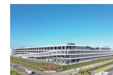
Exterior of DPL Nagareyama IV, a logistics facility covered by a disaster-prevention agreement
