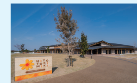
Cross-generational community center HITOTOKIMIKI in Miki City (Hyogo Prefecture)
