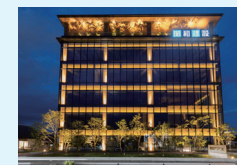
Head office building of SHOWA CONSTRUCTION CO., Ltd. (Fukuoka Prefecture)
